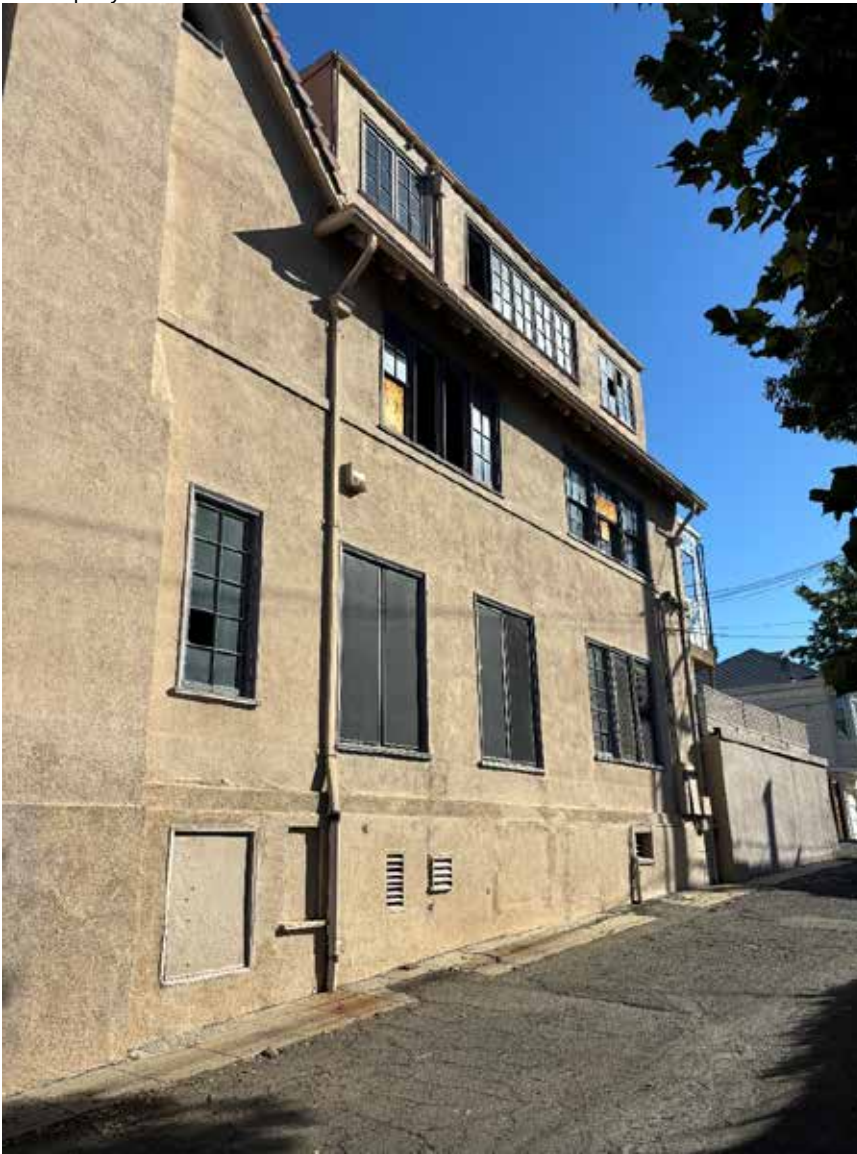
No. 004: South Elevation east massing, looking northeast.
